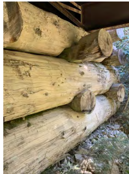
Left Bank Abutment when facing downstream
