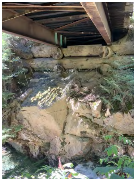
Right Bank Abutment when facing downstream
